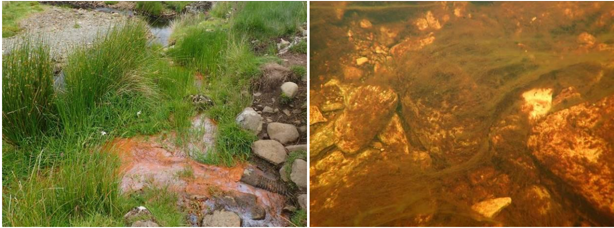
Plate 24. Land drainage outfall to the Elatagh River showing excessive iron-oxidizing bacteria.
